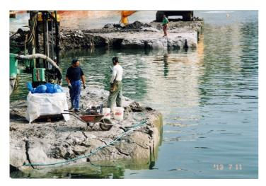
cement was opening in the pier. In the lower picture, taken the next day, the grab bucket removes the demolition waste generated afte the use of CRAS and the unnoticed but effective work done by this expansive agent in the demolition of a solid framework. CRAS performances are excellent in this type of work.
