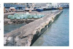
As a previous work to facilitate the CRAS application, several drillings have been carried out, 9 m deep and 70 cm in diameter. The upper picture shows the pier as it was prior to the demolition. The work in progress can be seen at the left picture, with the filling of holes with CRAS and the hollow that the breakage produced by the non-explosive demolition
